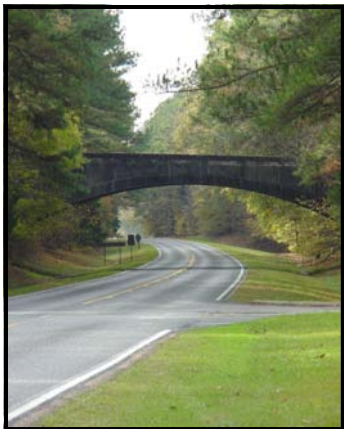
An overpass on the Natchez Trace Parkway—Nashville to Natchez.
